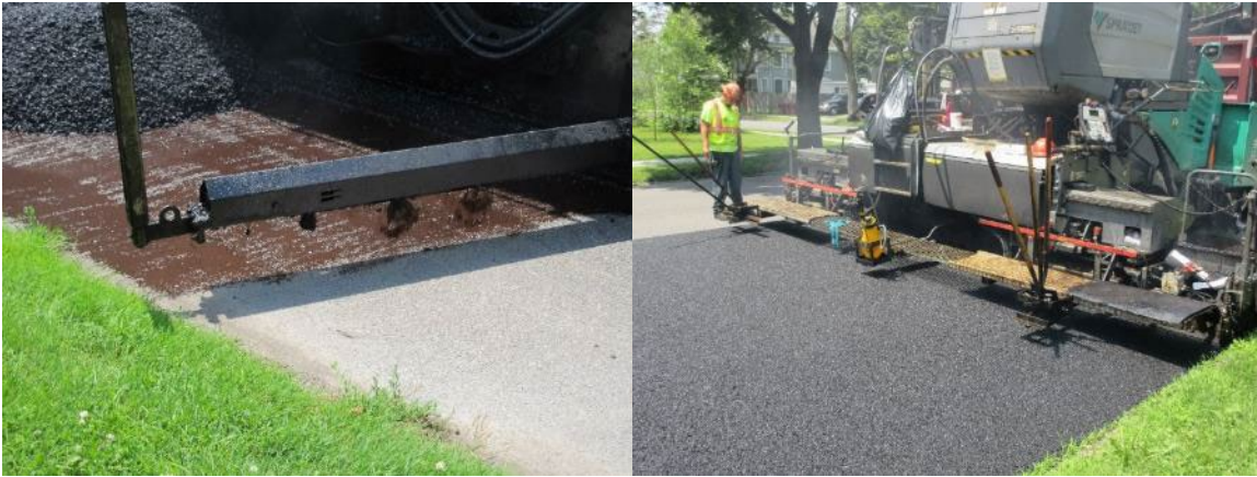
Figure 2 Emulsified asphalt being sprayed (left) and asphalt concrete being placed (right) in an UTBWC application (photos by Braham)
