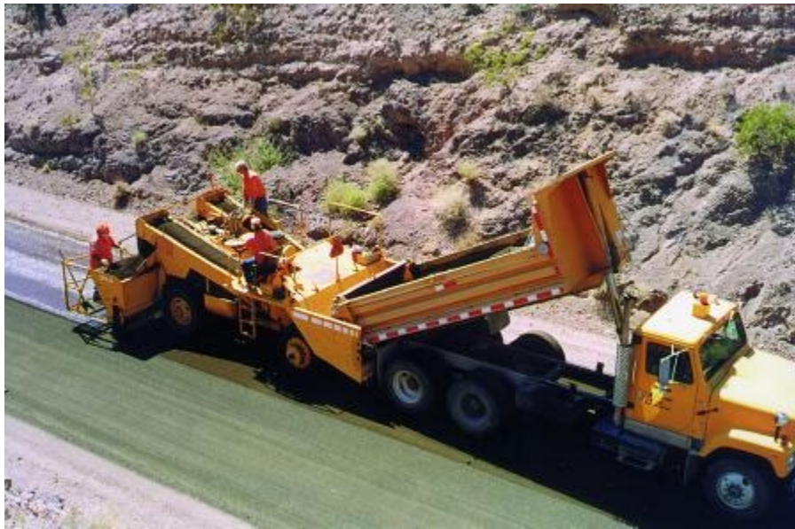
Figure 1 A sand seal being placed (Yamada, 1999)
